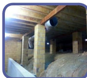
Sub Floor Ventilation
